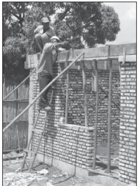
Pouring concrete for lintel at the Kamenge Clinic
